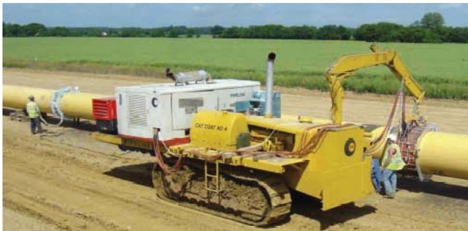
Figure 3.6 – Field applied joint coating (Source: http://www.pih.co.uk/uploads/files/fusion_bonded_epoxy.pdf )
