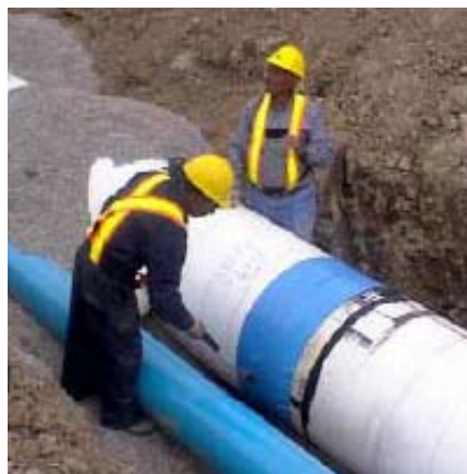
Figure 3.7 – Shrink sleeve application (Source: http://www.covalencecp.com/documentos/casos/JR-013-WaterWrap.pdf )
