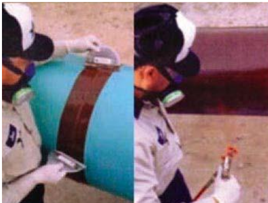
Figure 5.5 – Powercrete® pipeline coating application ( http://www.petropages.com/vendors/v19548.htm )
