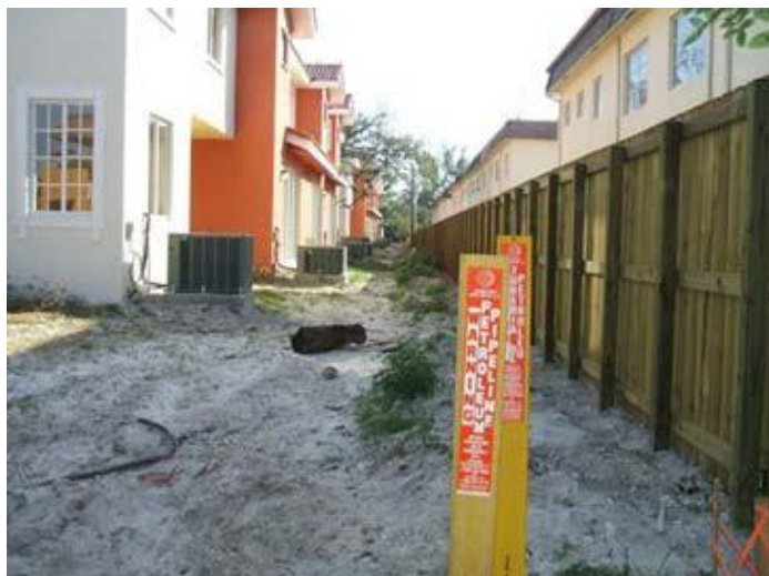
Figure 5.1 – Pipeline encroachment in residential development. http://www.apga.org/library/PHMSA%20notices/PIPA_Flier_Final.pdf
