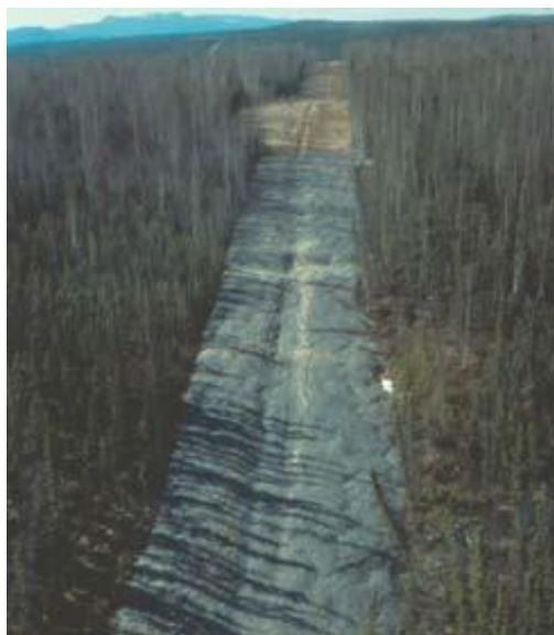
Figure 5.9 – Illustration of a cleared right-of-way along a pipeline route
