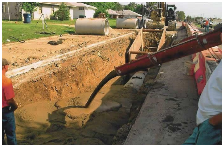
Figure 5.8 – Flowable fill being poured to fill the pipe excavation area. ( http://www.irmca.com/Topics/flow.asp )
