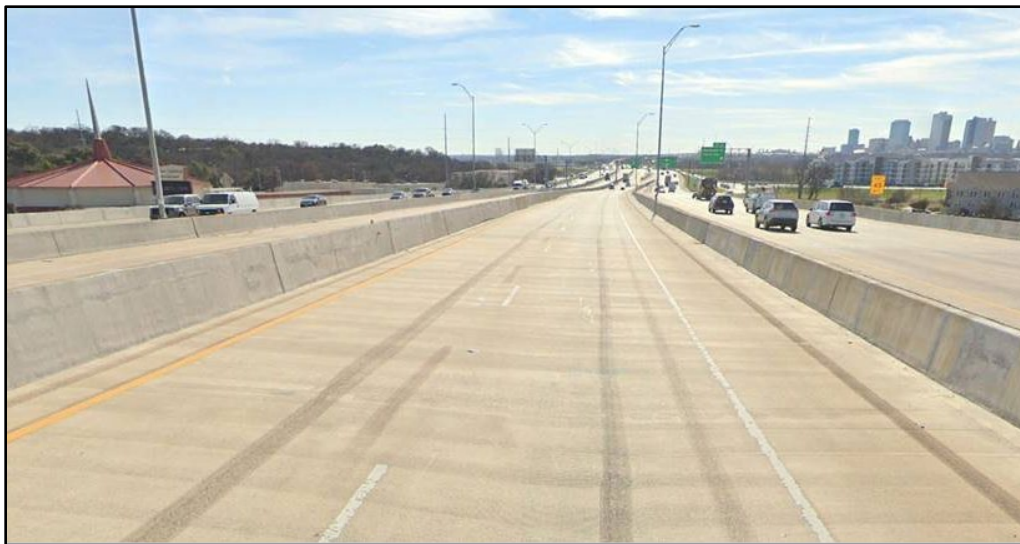
Figure 1. Approximate location of crash, looking south. (Source: Google Earth image from January 2020)
